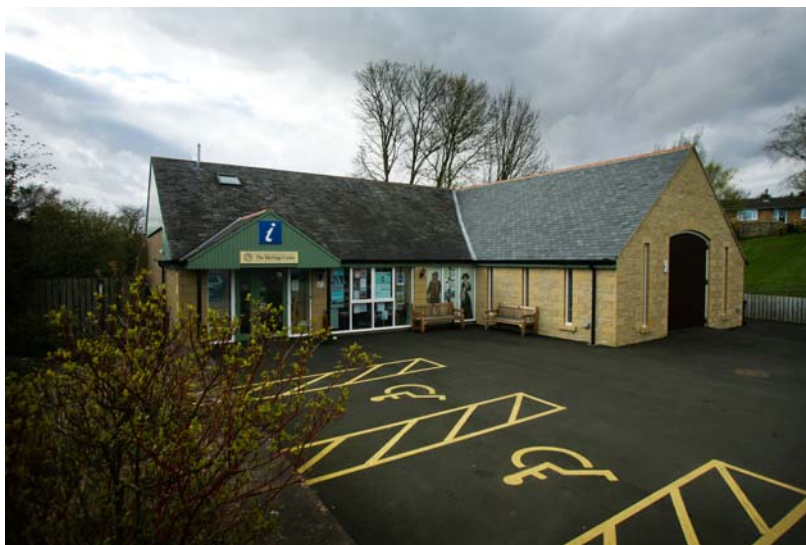
The Heritage Centre and TIC
